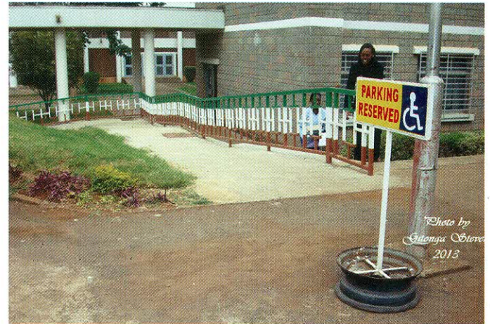
Ramp and reserved parking bay for PWDs at KEFRI headquarters
