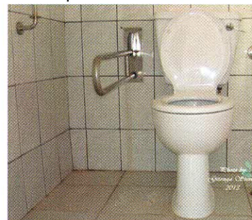
Disability friendly toilet at KEFRI head office
